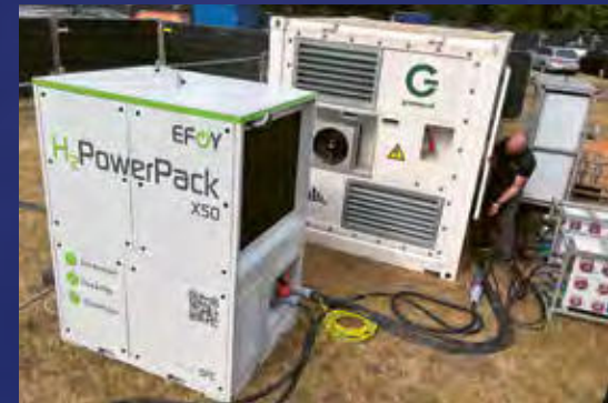
Set up with the fuel cell that loads the battery pack
