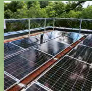
The photovoltaic system has an output of 5 kWp
